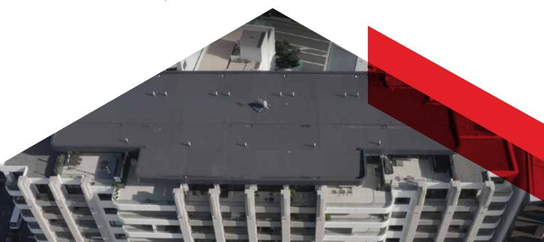
Our system build up has been thoroughly and independently tested and has demonstrated an average uplift of 14kpa, well above building code requirements.
