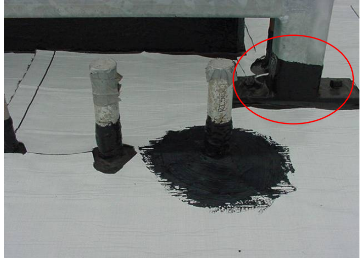
▲ Circled area shows instance of LDC membrane detailing applied to metal up-stand along with M-2000 detailing to pipe penetrations in foreground.
