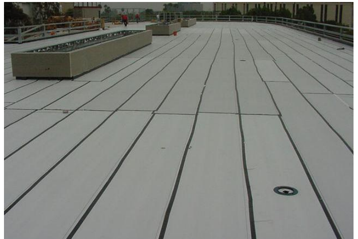
▲ Plaza deck drain detailed with 2.3mm layer of Volclay M-2000
