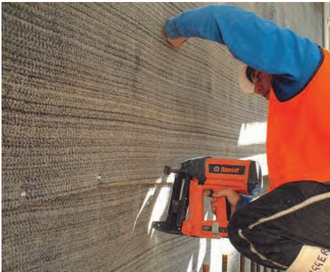
▲ Application of Volclay® at the Auckland War Memorial Museum With the use of modern fastening techniques, installation of the membrane is quick and straight forward in any weather condition.
