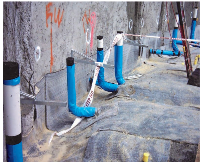
▲ Numerous pipe penetrations, for drainage and services are detailed with Volclay® Waterstoppage (granular bentonite). Bentoseal® and Waterstop-Rx® were used on larger penetrations.
