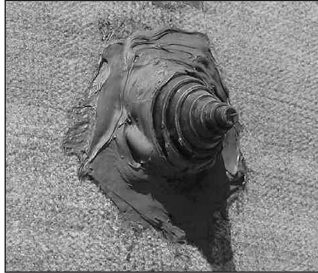
Volclay TB-Boot installed over soldier pile tie-back head with Bentoseal applied around the base perimeter of the boot and onto the Voltex DS membrane.
